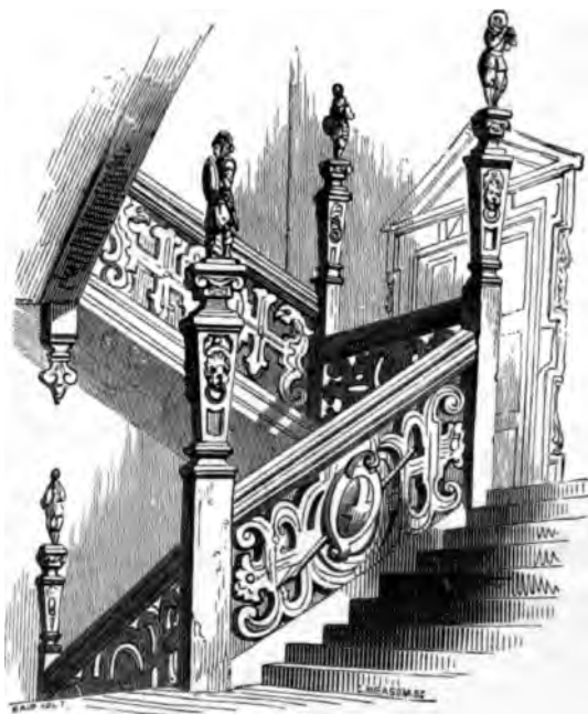
STAIRCASE IN GENERAL IRETON'S HOUSE, DATED 1630.
